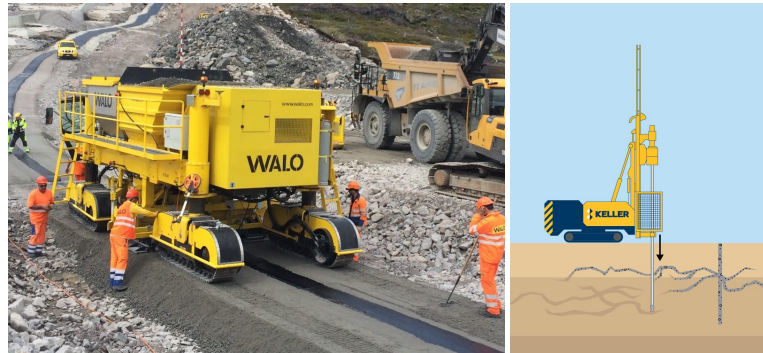
Figure 1.10. – Example of artificial cemented granular soils: Asphalt core dam, cement grouting soil improvement. Reference: https://walo.com .
